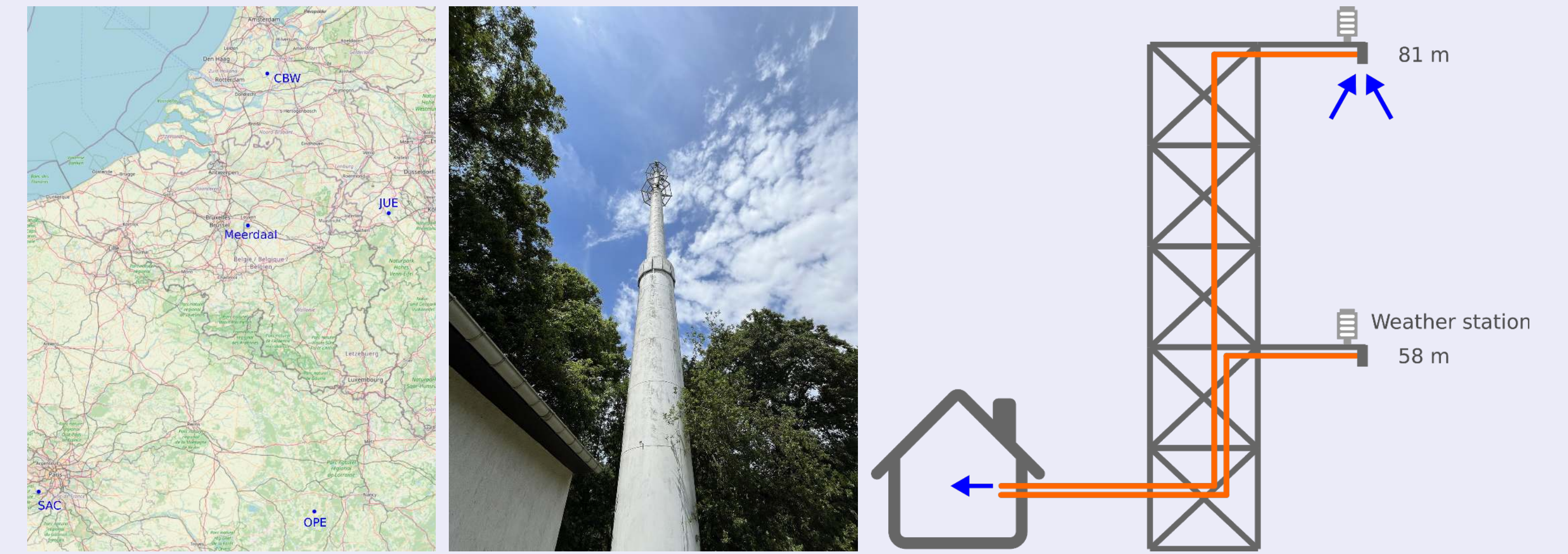
Figure: Left: Location of Meerdaal and the surrounding ICOS stations. Middle: The communications tower in Meerdaal with the two platforms at 58 and 81 m. Right: Diagram of the tower measurement setup.
